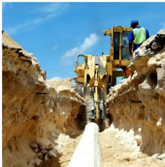
*Installation of a potable water distribution pipeline in the Cayman Islands
